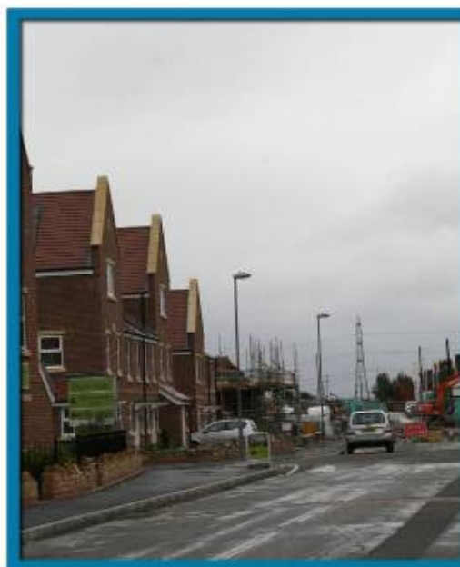
FIGURE 11.1: SHIREBROOK MODEL VILLAGE DEMOLITION AND PLACE SHAPING ACTIVITY ON-SITE 2010
