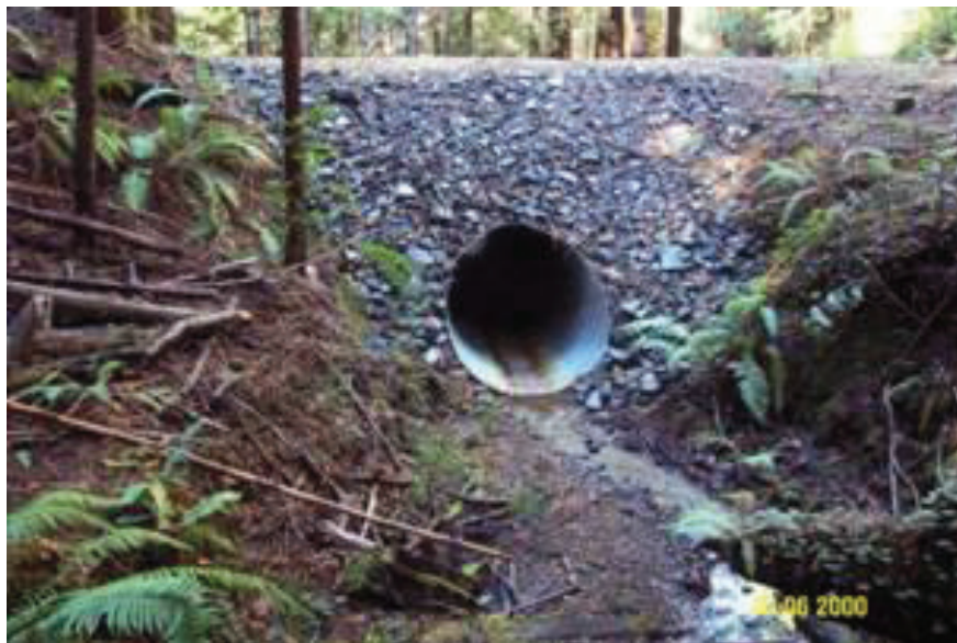
Figure 9: Typical culvert crossing
