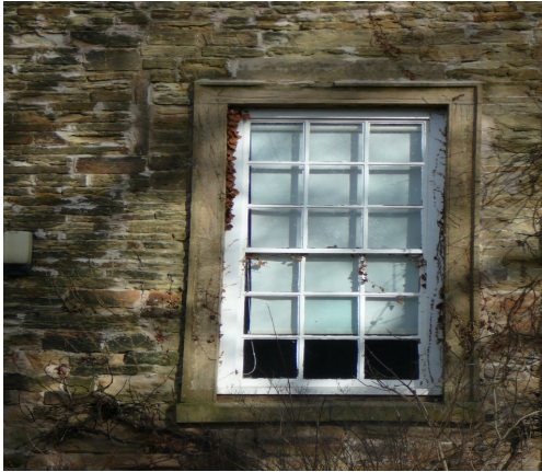
Georgian-style sash window
