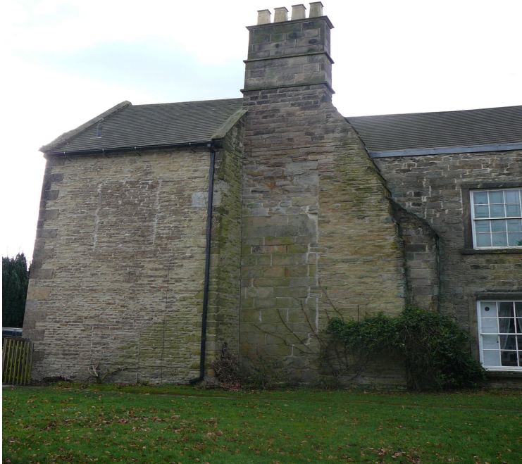
A main chimney stack at Carnfield Hall which has been extended twice
