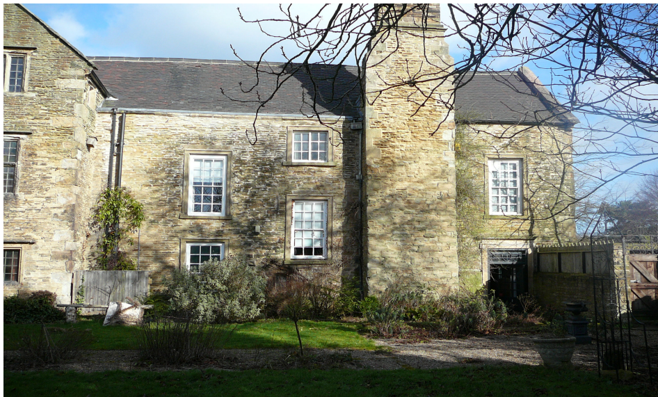
Carnfield Hall – part of the south elevation
