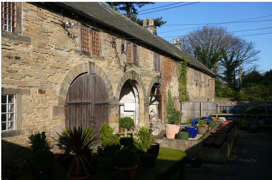
The former coach house showing the three central arches (east elevation)
