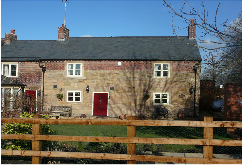
Carnfield Wood Farm – note the brick course under the eaves.
