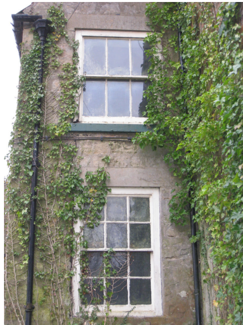
Twelve and six-pane sliding-sash windows at Springfield Farm
