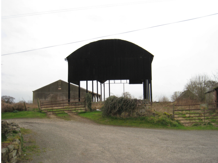
Barns to the south of Mill Wood Lane
