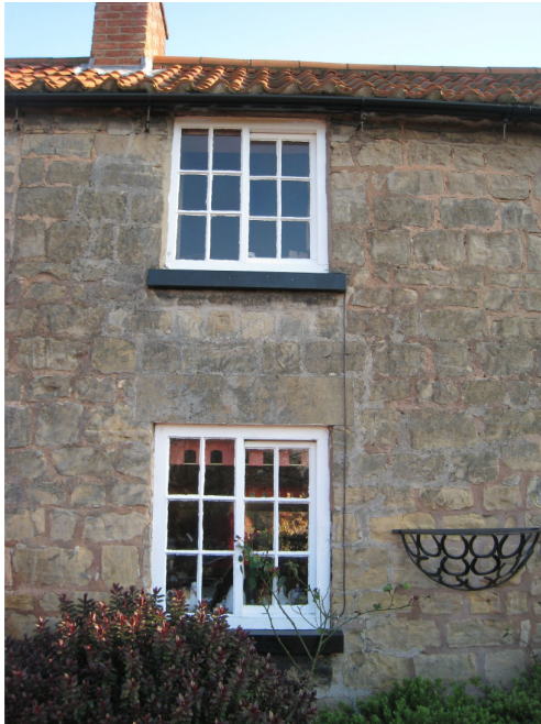
Horizontal sliding sash windows with projecting sills
