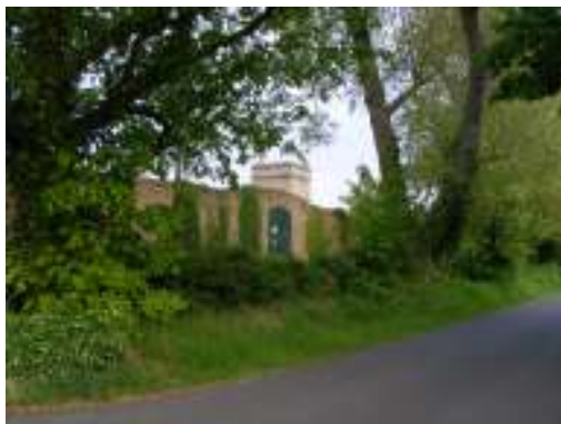
Water Tower and Shed
