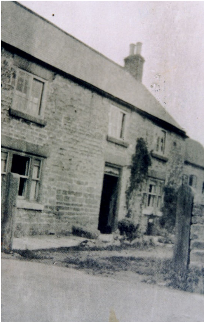
Undated photograph of vertical and horizontal sliding sash windows at Forest Cottage (courtesy of Ivor Milnes).
