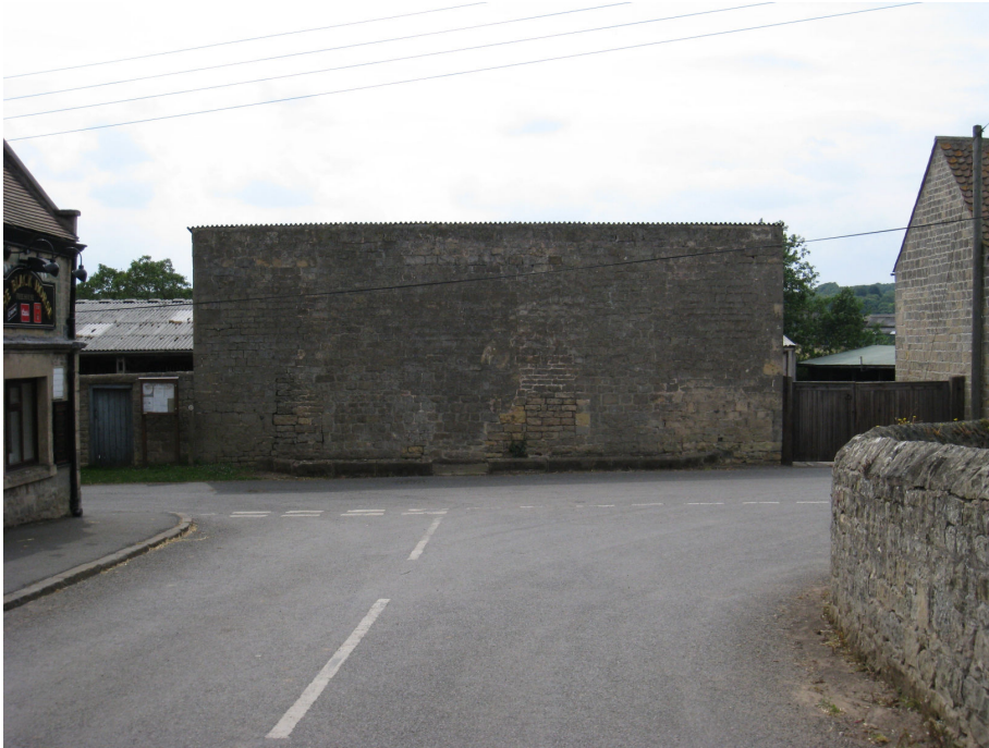
Former farmhouse at Whaley Moor Farm
