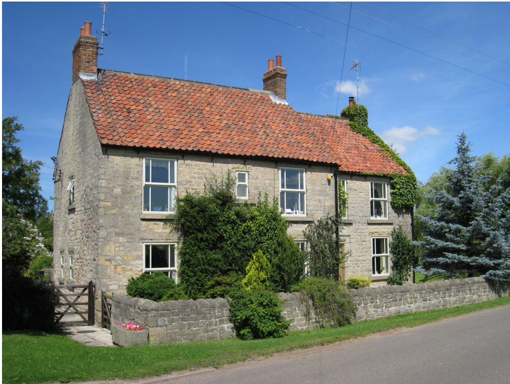
Pinewood Cottage built in the local vernacular style; constructed of magnesian limestone with pantile roof, brick chimney stacks at gable end and cast iron rainwater goods (20 th century extension to right)
