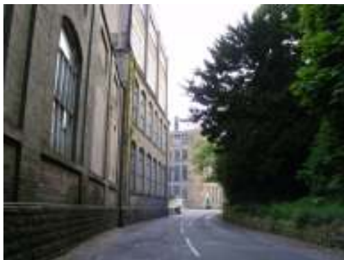
Mill Chimney (part)
