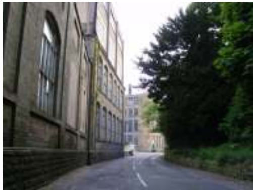
Mill Chimney (part)
