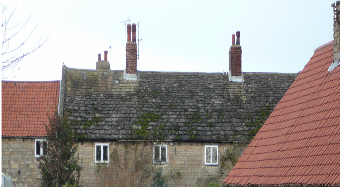
Contrast in roofing materials between Steetley Farmhouse and other buildings
