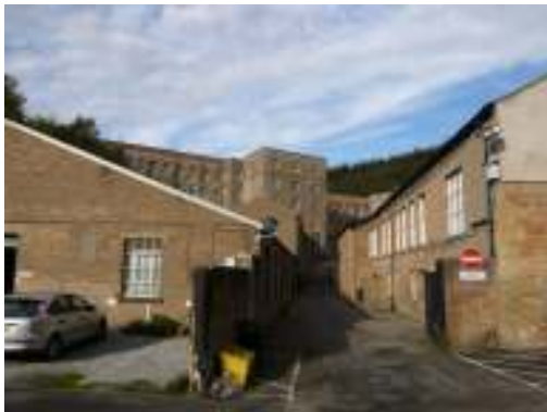
Rear of Mill 2
