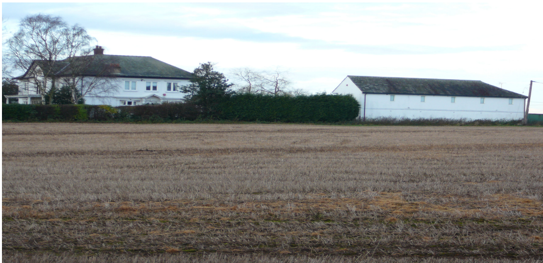
Steeley House and adjacent outbuildings
