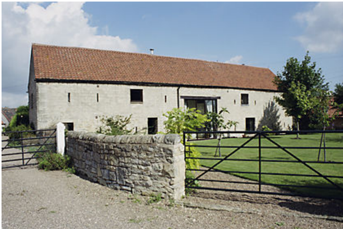
The Barn at Steetley (photograph courtesy of English Heritage)
