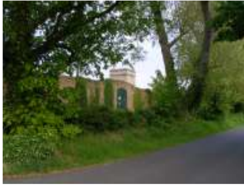
Former Warehouse and Water Tower
