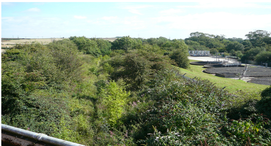
Former railway line north of Hollinhill Grips – overgrown and impassable
