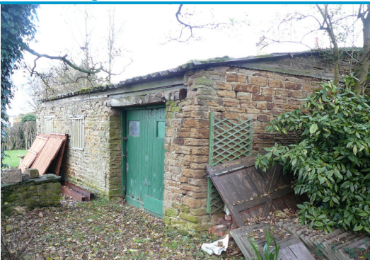
The former smithy, Craig House – stone and originally pantiled roof, although now has a replacement corrugated sheet roof
