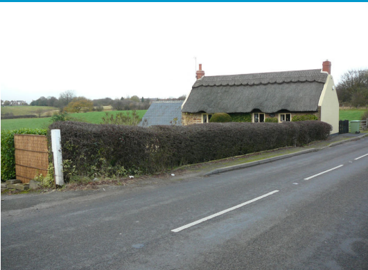
Devonshire Cottage, Cragg Lane – stone and thatched cottage dating from the late 1700s. Recently extended with rendered gables.
