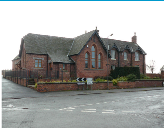
The Old School, Huthwaite Lane – former school converted in 2006 to two residential properties. Red brick and slate with a range of interesting detailing including gothic style windows
