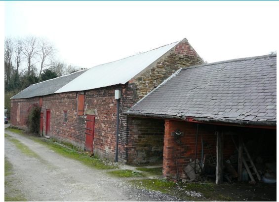
Traditional outbuilding range, Church Hill Farm – red brick and slate, with replacement corrugated sheet in places. May be contemporary with the farmhouse
