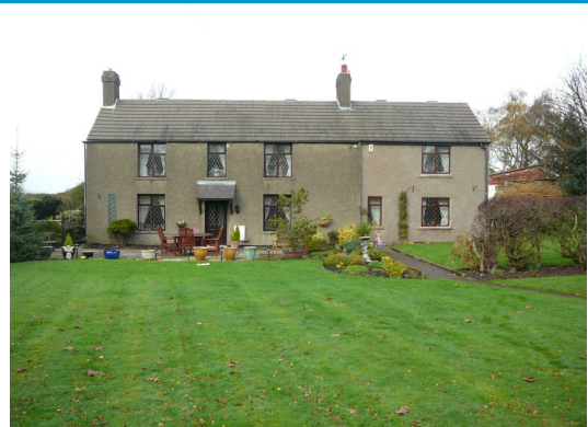
Craig House, Cragg Lane – two-storey extended cottage; rendered with concrete tiles. Dating from the early 1800s
