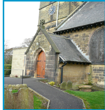
The south porch
