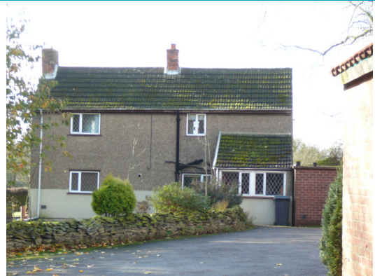
The Cottage, Pipes Farm – rendered facades with concrete tile roof and modern windows
