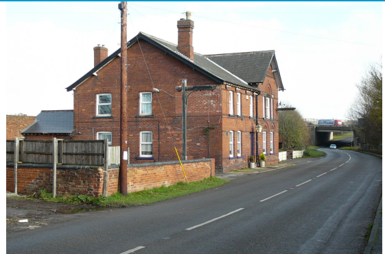
The former Robin Hood Hotel – view looking east with the M1 motorway running along the edge of the conservation area
