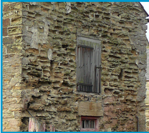
Examples of eroded Coal Measures sandstone and a rendered façade
