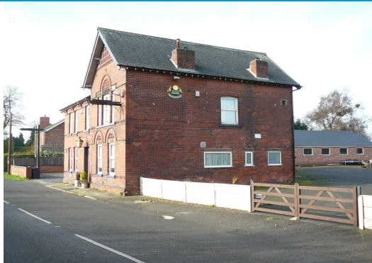
The Robin Hood Hotel - substantial late Victorian former public house. Red brick and slate with a range of interesting detailing. Modern windows.
