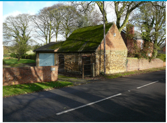
Outbuilding at Old Farm Cottage, Huthwaite Lane – stone and brick with corrugated sheet roof
