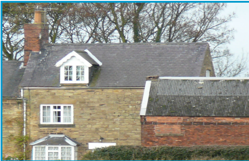
An assortment of different building materials, Church Hill Farm
