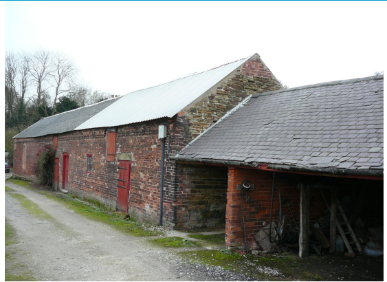
Traditional outbuilding range, Church Hill Farm – red brick and slate, with replacement corrugated sheet in places. May be contemporary with the farmhouse
