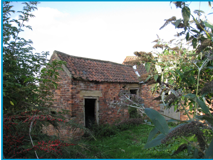
Former cow shed to the rear of Wayside
