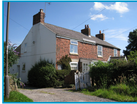
Re-fronting in brick and rendering at Pentuan Cottage and Poplar Farm Cottage
