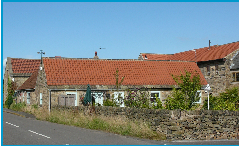
Clay pantile roofs of converted farm buildings on Deep Lane, some have eaves course of stone slate and stone coped gables
