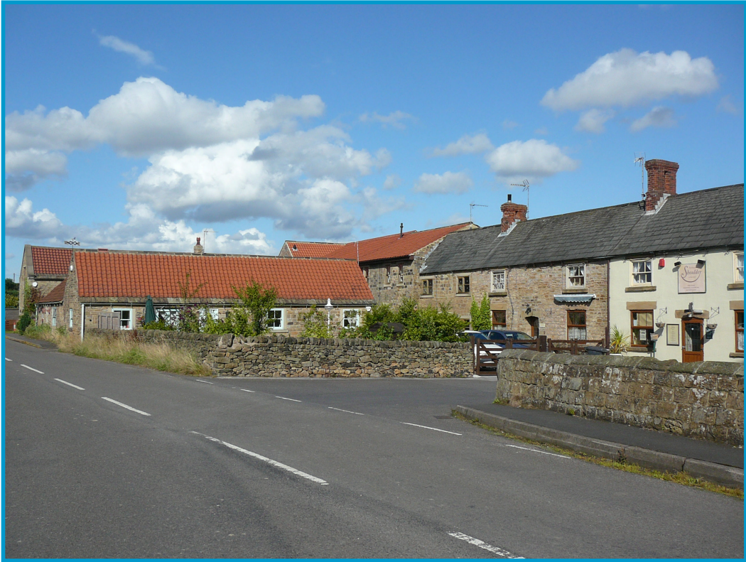
View of The Famous Shoulder public house and converted barns and outbuildings
