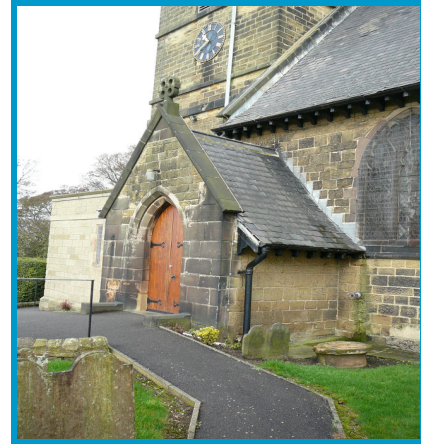
The south porch
