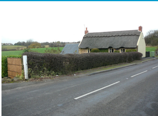
Devonshire Cottage, Cragg Lane – stone and thatched cottage dating from the late 1700s. Recently extended with rendered gables.
