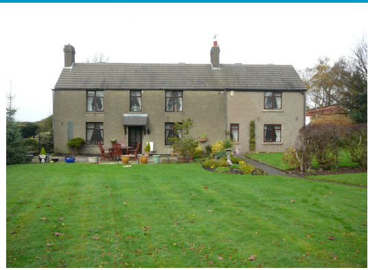
Craig House, Cragg Lane – two-storey extended cottage; rendered, with concrete tiles. Dating from the early 1800s
