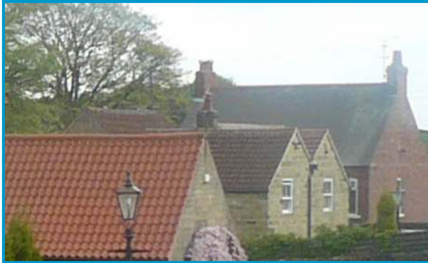
Variety in the type of roofing materials
