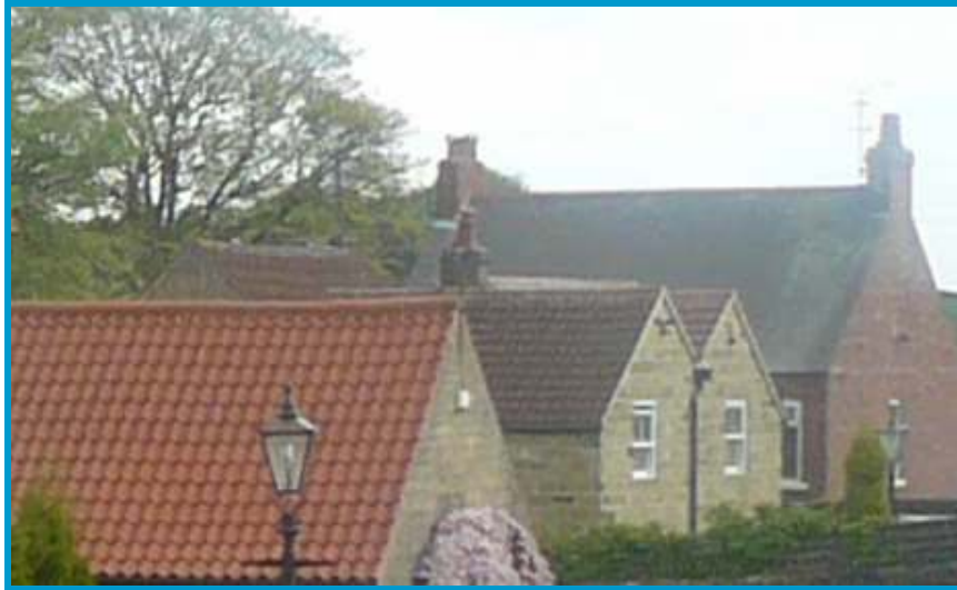
Variety in the type of roofing materials
