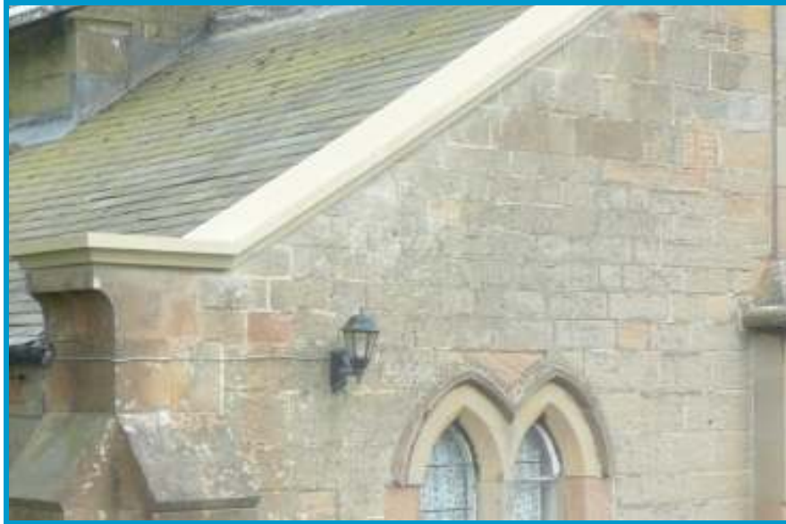
Evidence of modern stone repairs, Church of St Leonard
