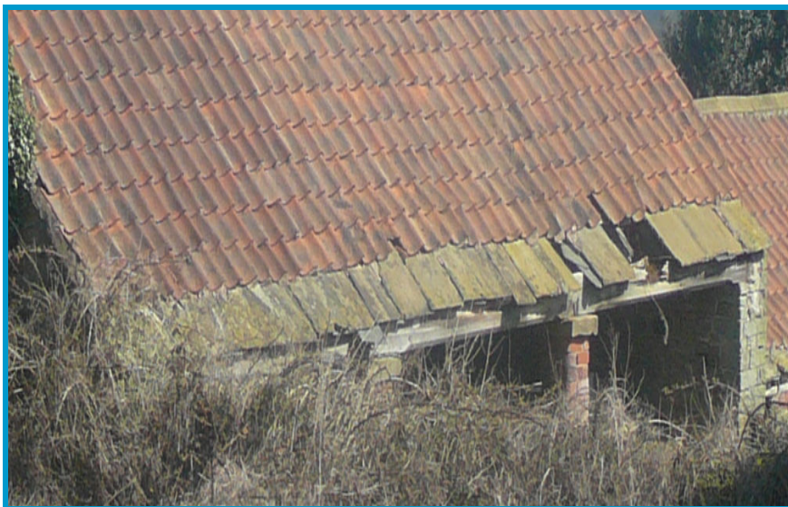
Pantile roof with stone slate eaves course
