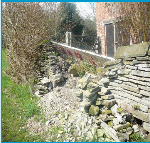
Examples of stone walls requiring repair
