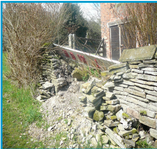
Examples of stone walls requiring repair
