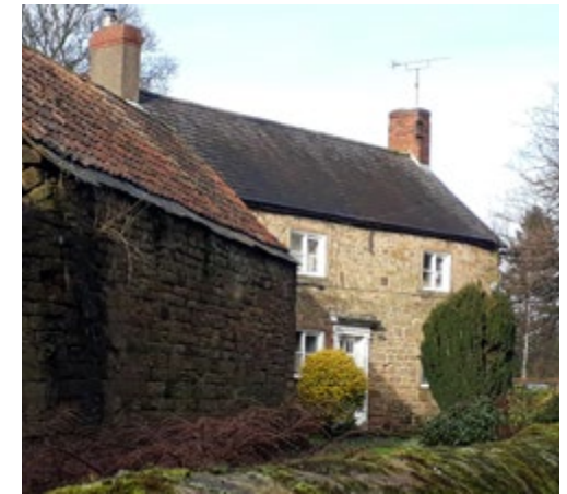
Traditional windows and doorcase, Stainsby
