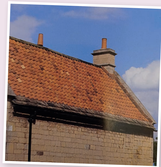
Pantiles at Bolsover. The two course of stone slates gives stronger eaves with better projection from the wall.
