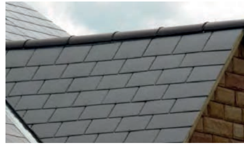
Slate roof with a thin leading edge profile provides a high quality finish.
