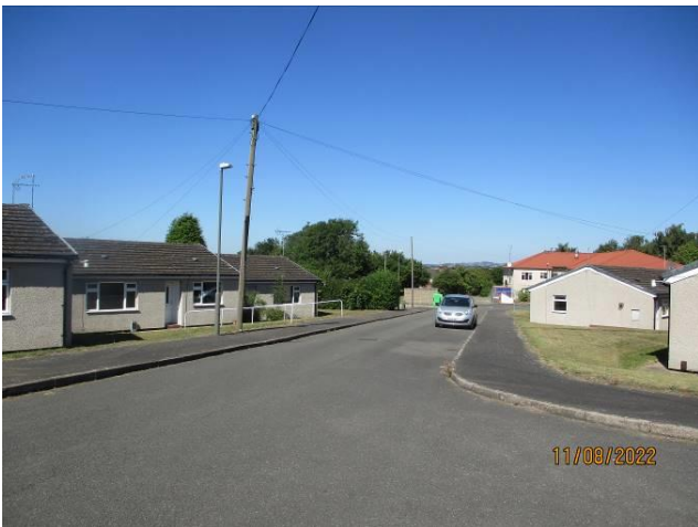
Views within Woburn Close of existing bungalows
