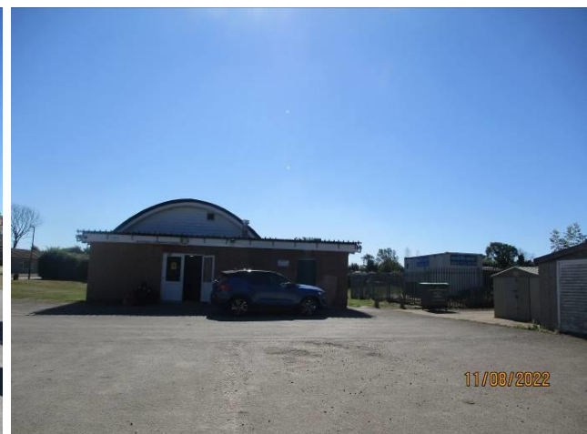
View of existing Community Centre
