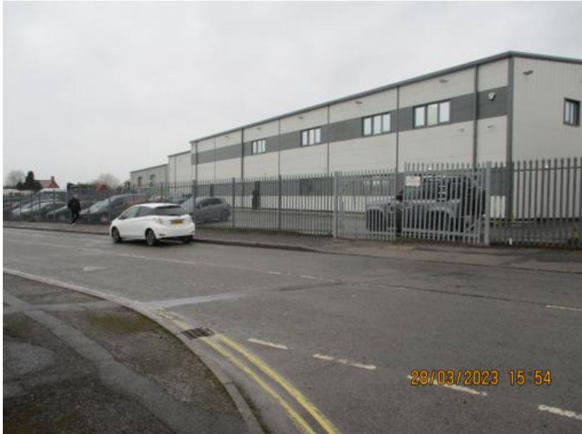
The adjacent unit which demonstrates the proposed steel cladding and colour of the proposed development for its elevations and roof.
