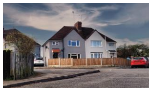
Improving the thermal performance of 92 existing dwellings
