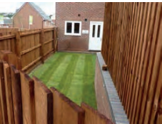
Cramped gardens are unsuitable for family accommodation.
