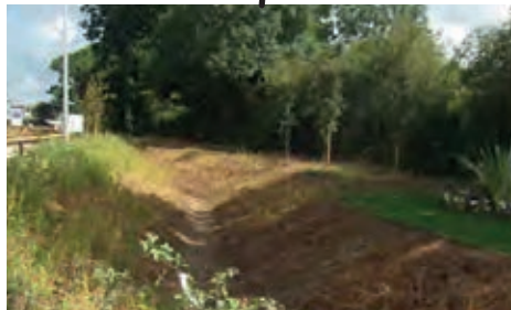
SuDs swales in a green corridor
