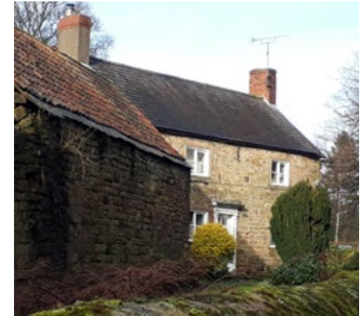
Traditional windows and doorcase, Stainsby
