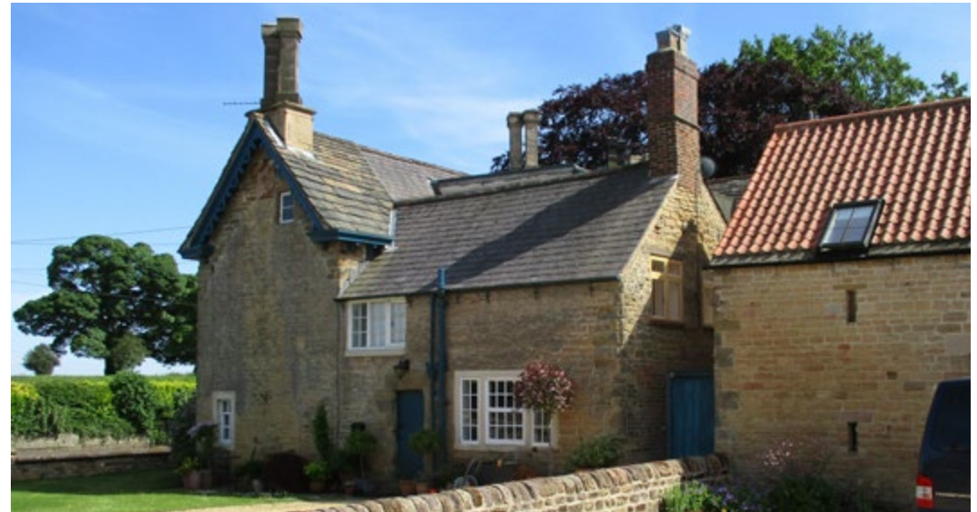
Oversailing eaves with barge boards, Hardwick and Rowthorne
